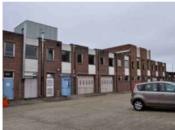
Rear view of site
